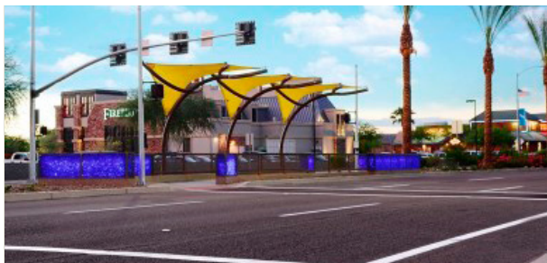
HAWK or High-intensity Activated crosswalk -- provides a protected pedestrian crossing in Scottsdale.
