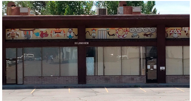
Vacant properties along Longview Drive within the White Rock Town Center.
