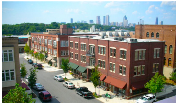
Downtown housing designed to fit into the traditional downtown character.
