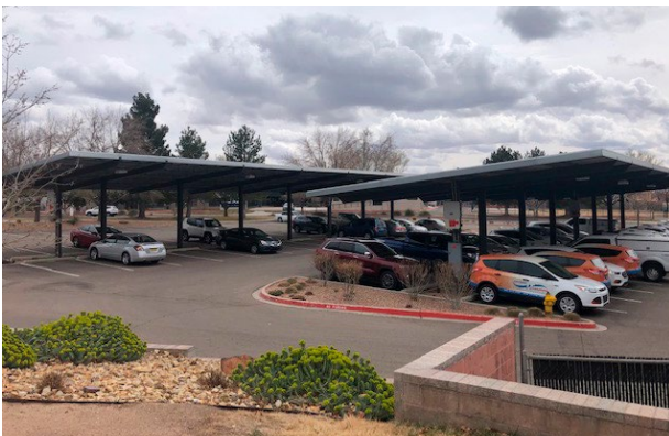
Solar covered parking in Albuquerque, NM
