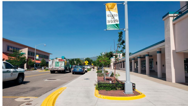
Existing improvements along Central Avenue
