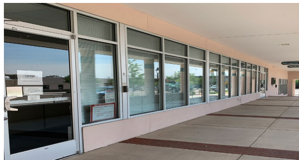
Ground floor office uses along Central Avenue create inactive store fronts
