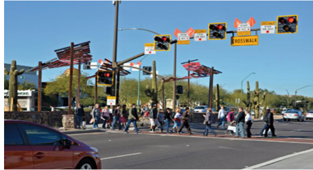
HAWK or High-intensity Activated crosswalk -- provides a protected pedestrian crossing in Scottsdale.
