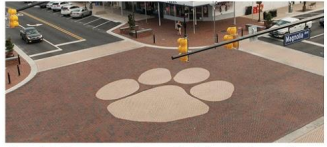
Speed-tables or varying materials at intersections as placemaking and to enhance pedestrian safety
