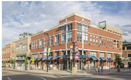
Parking structure with mixed-use liner building in Albuquerque
