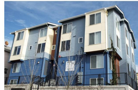
Solana Suites, Seattle, WA: 36 units, 11,100 SF
