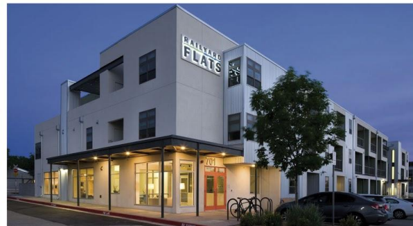
Railyard Flats, Santa Fe: approx. 45,000 SF
