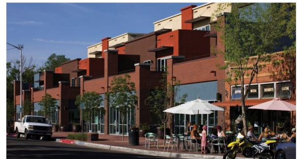
Bricklight Courtyards, Albuquerque: MF, retail - 42,000 SF
